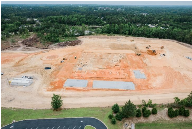
Drone photo of the construction site on the day of the groundbreaking, May 25, 2022.
